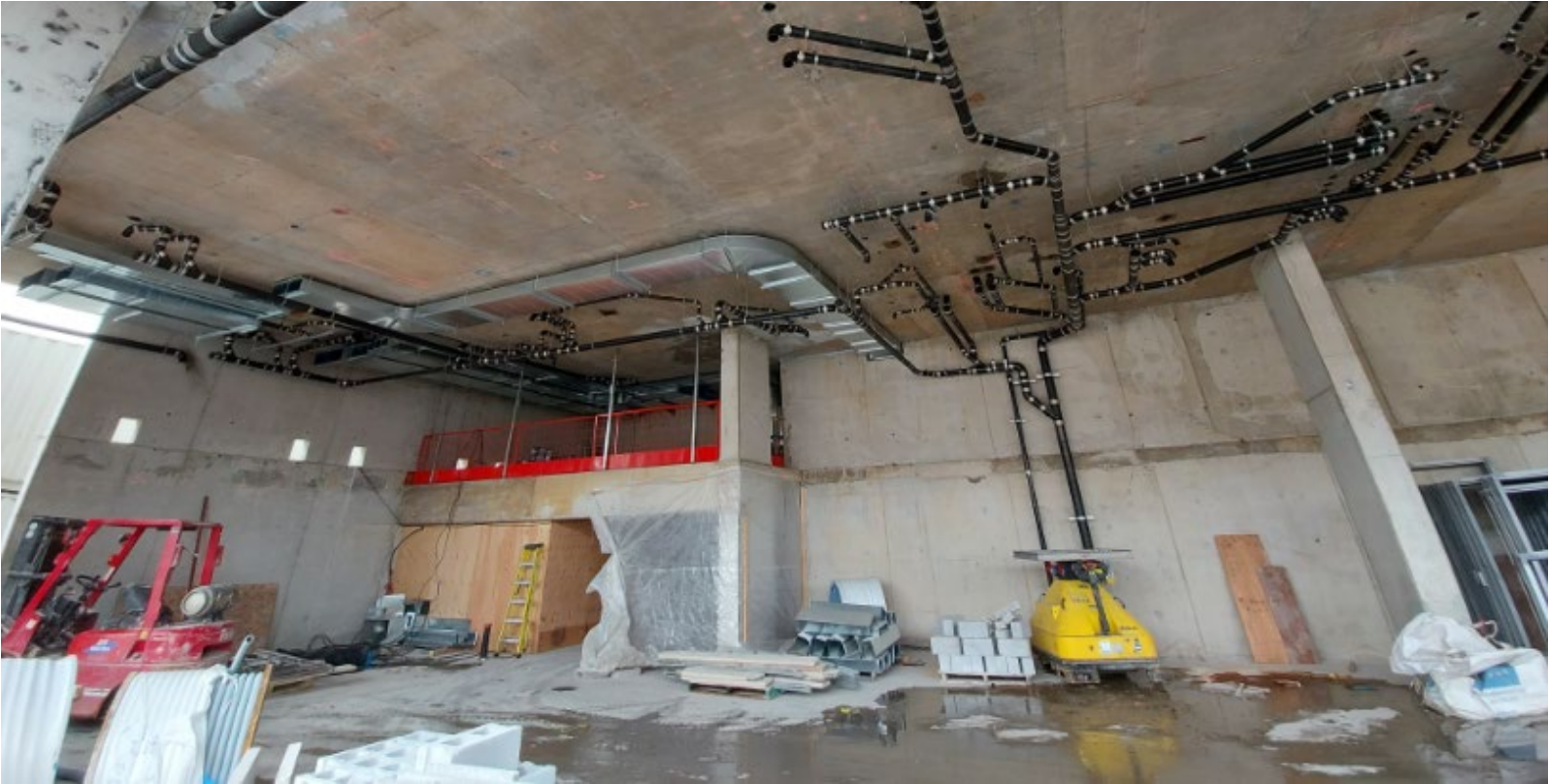
View of the teen area, hallway to the washrooms, and the program room
