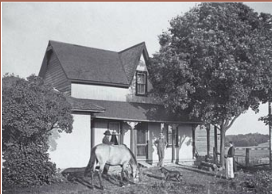
Scarborough past: The William Chester house and residents, at the north-east corner of Ellesmere Road and Morrish Road, photographed in 1908, by Joseph A. Blakey — well before the 20 th century suburbanization of Scarborough. This picture is part of a permanent display highlighting the local history collection at Cedarbrae District Branch. The original photograph is part of the Canadian Historical Picture Collection at Toronto Reference Library.
